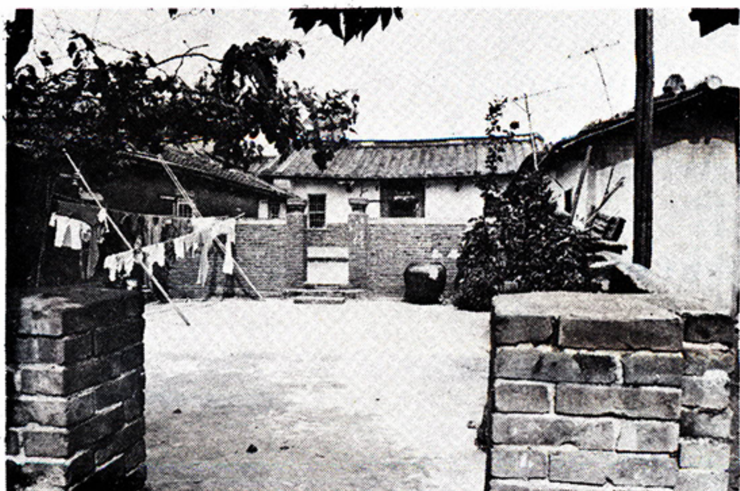
船頭巷二九號楊宅
